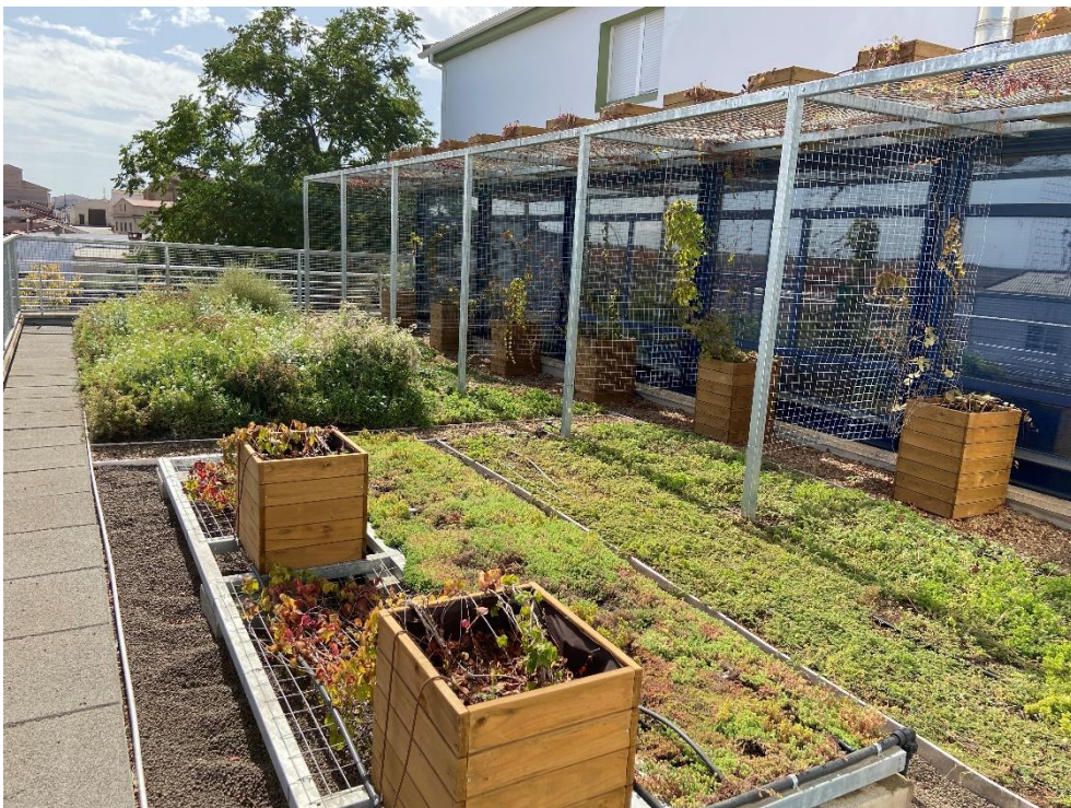
One of the green roofs implemented in the project (mBiGCUVE 2 prototype)
