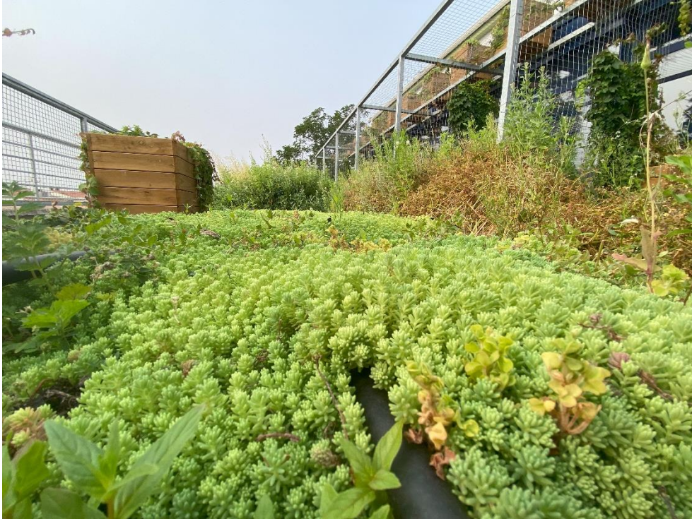
View from one of the green roofs implemented in the Gabriela Mistral primary school
