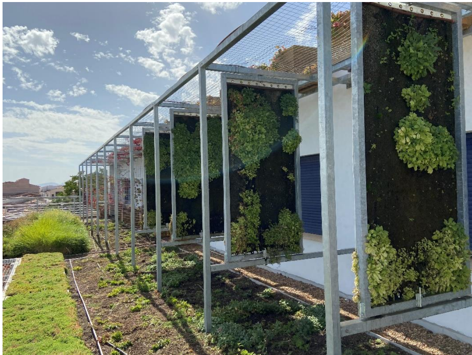
One of the green facades implemented during the project (prototype mBiGToldo)
