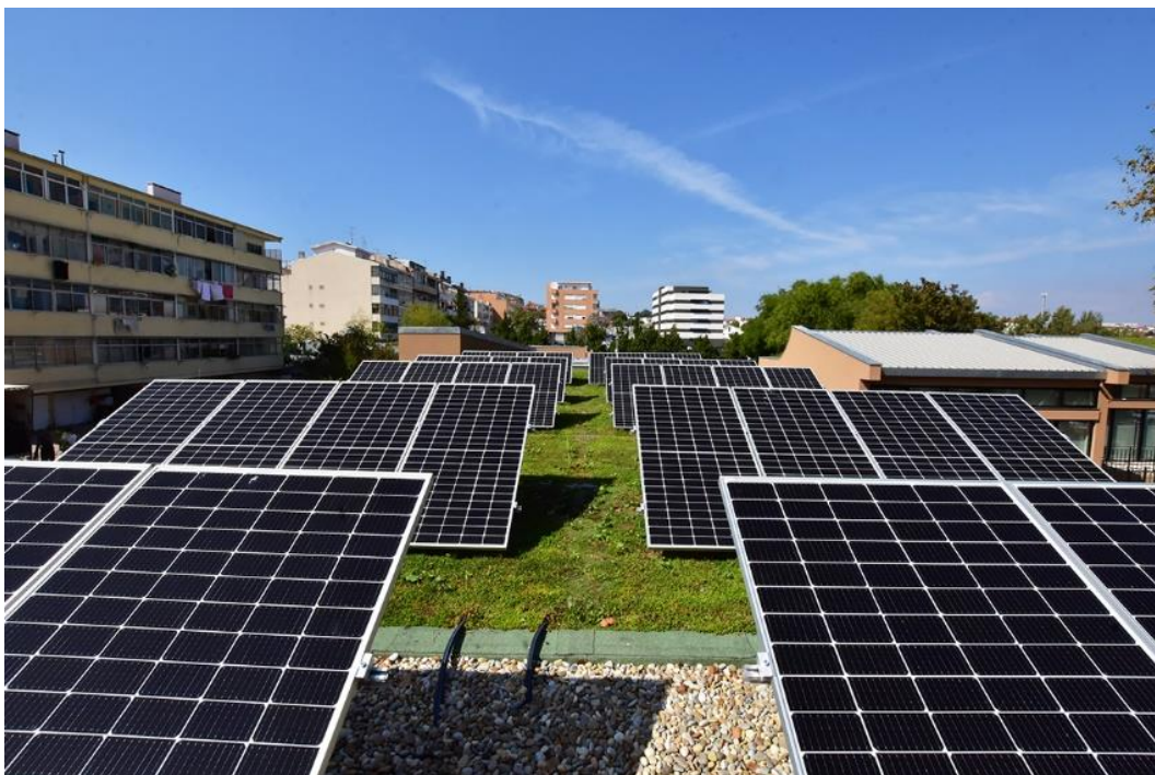
One of the green roofs implemented in EB1 Falcão
