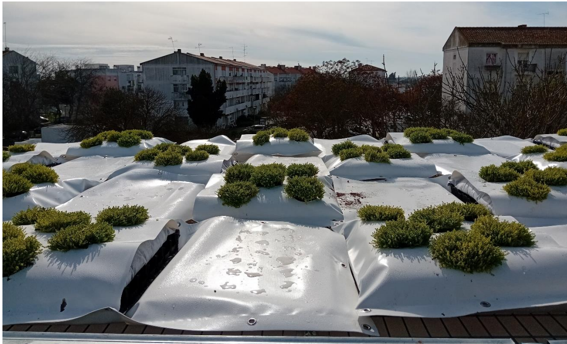
Green roof implemented at EB1 Horta das Figueiras
