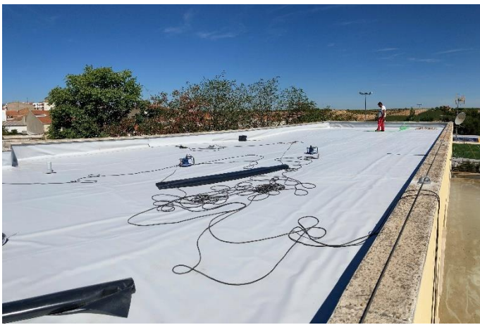
Figure 1 Application of PVC film waterproofing.
