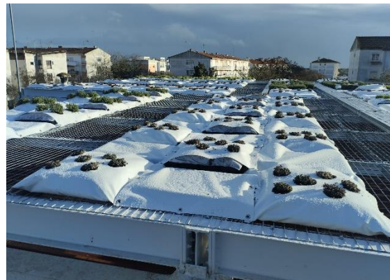
Figure 24 Green roof. mBIGWTray prototype.
