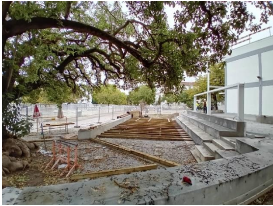
Figure 29 Permeable exterior paving. Installation of a suspended wooden platform.
