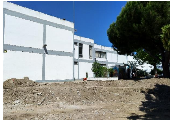
Figure 19 East façade before NBS implementation.
