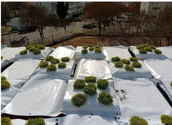
Figure 25 Green roof. mBIGWTray prototype.
