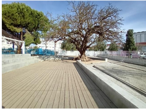
Figure 30 Permeable exterior flooring. Suspended wooden platform.
