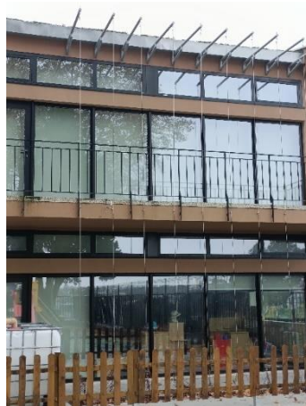
Figure 39 Steel cable structure.
