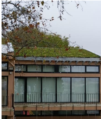
Figure 38 mBiGUL prototype - sloping roof.
