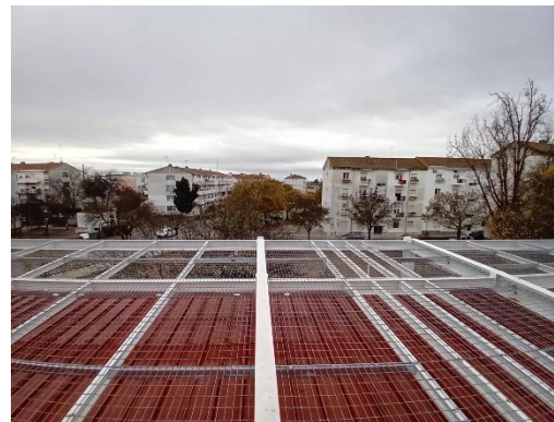
Figure 23 Metallic structure. Roof.
