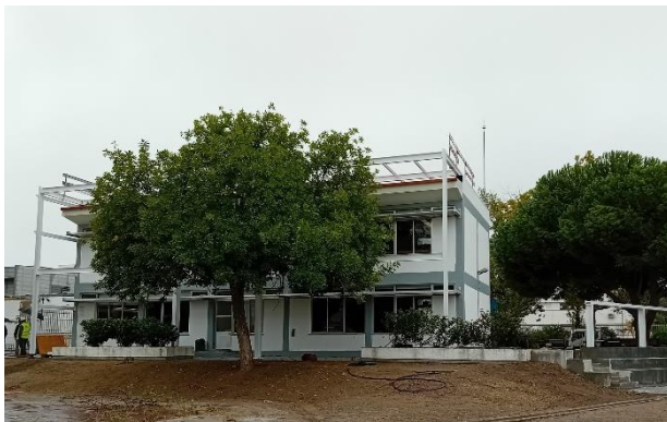
Figure 22 Metallic structure. South façade.
