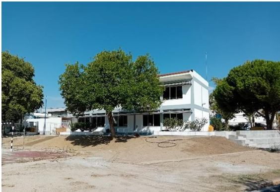
Figure 18 South façade before NBS implementation.
