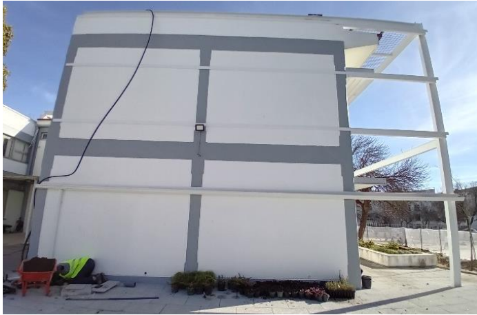
Figure 26 West façade. Installation of metal structure to support the mBIGToldo prototype.
