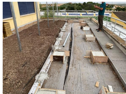
Figure 4 Implementation of "cold roofs".
