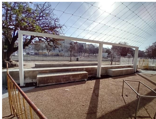
Figure 28 Steel cable structure.
