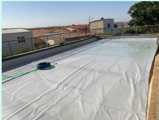
Figure 15 Waterproofing test by flooding.
