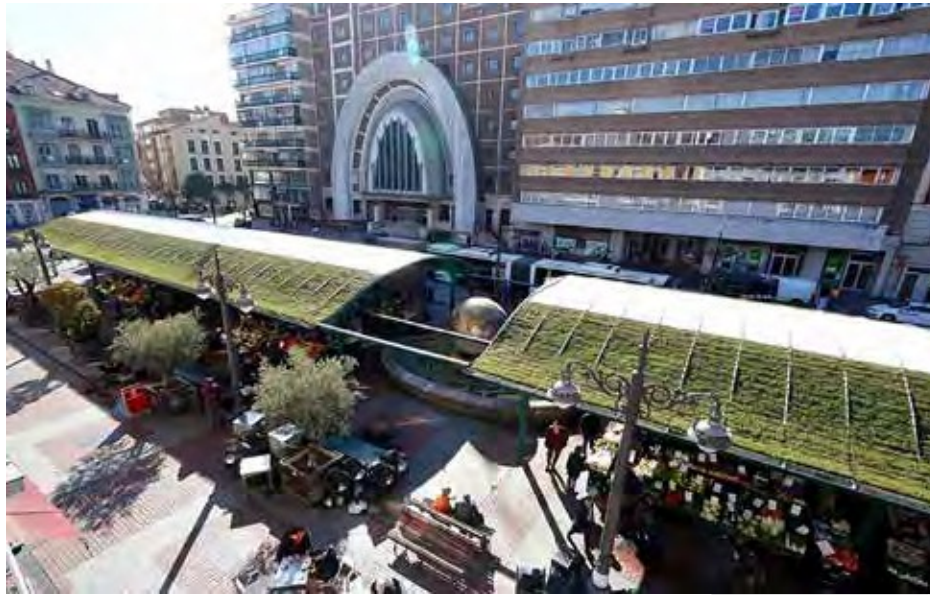
Figure 5. Green roof on the canopies of Plaza España in Valladolid (Source: Valladolid City Hall).
