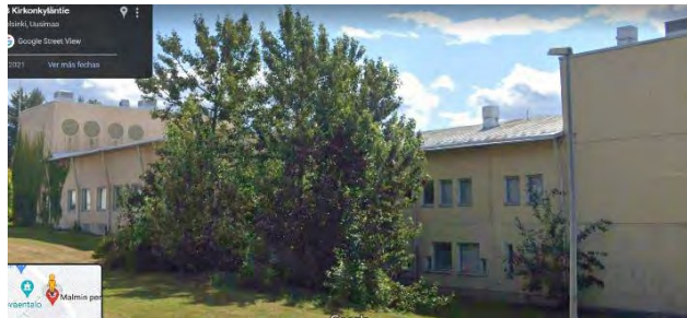
Illustration 58. Northwest façade (Malmin Elementary School)
