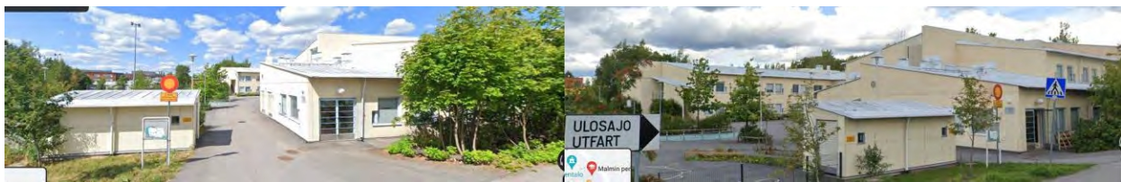
Illustration 60. Southwest façade (Malmin Elementary School)
