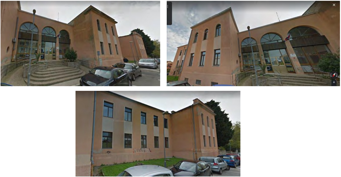
Illustration 33. North façade (Stoja Primary school, Pula, CROATIA)
