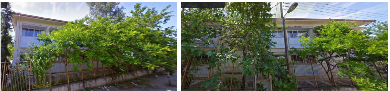
Illustration 49. Northwest façade (5th High School of Peristeri)
