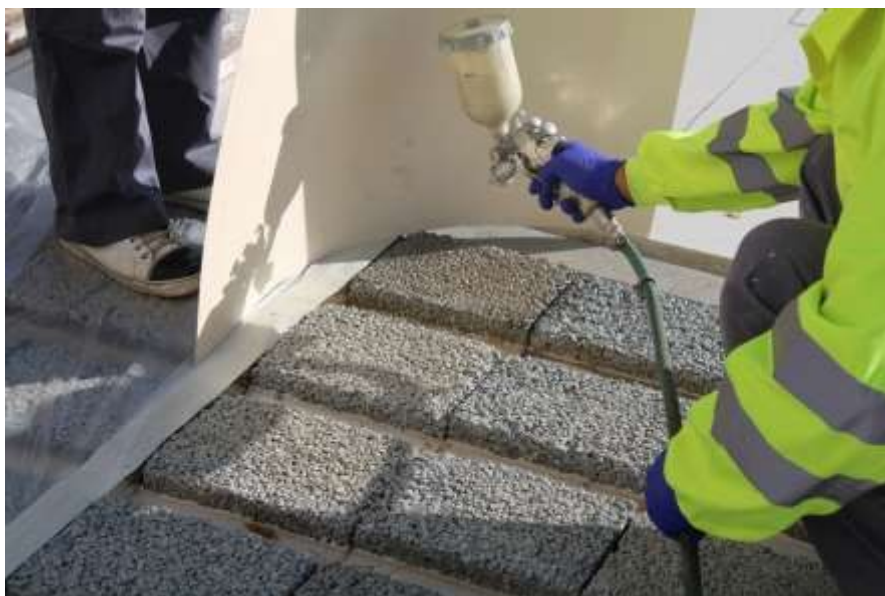
Figure 17: Application of the photocatalytic emulsion.
