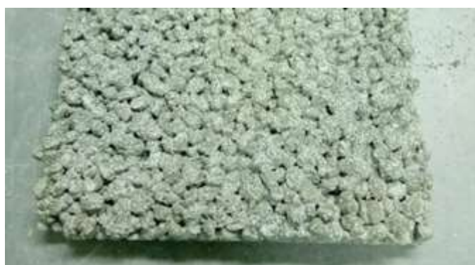
Figure 12: Final surface appearance of the selected porous concrete.
