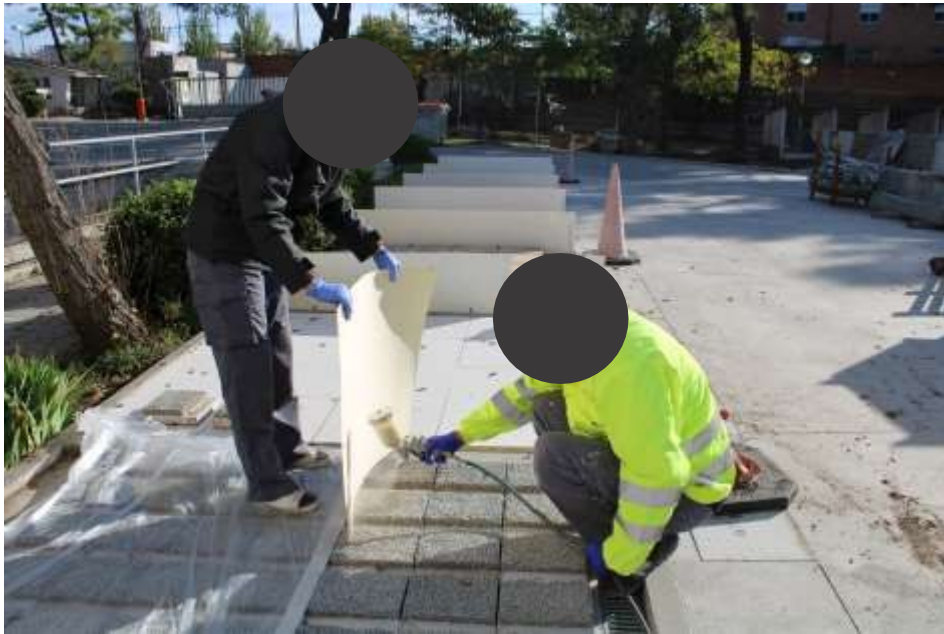
Figure 18: Application of the photocatalytic emulsion.
