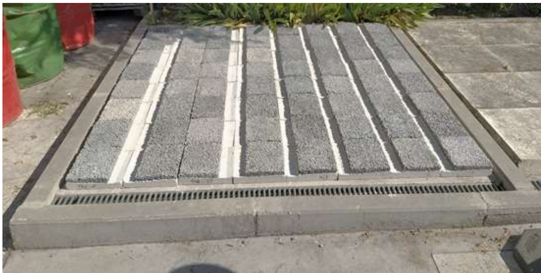
Figure 15: Tiles installed in the IETcc-CSIC facilities.
