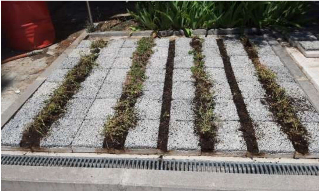
Figure 16: Pavement with vegetation installed on the IETcc-CSIC platform.
