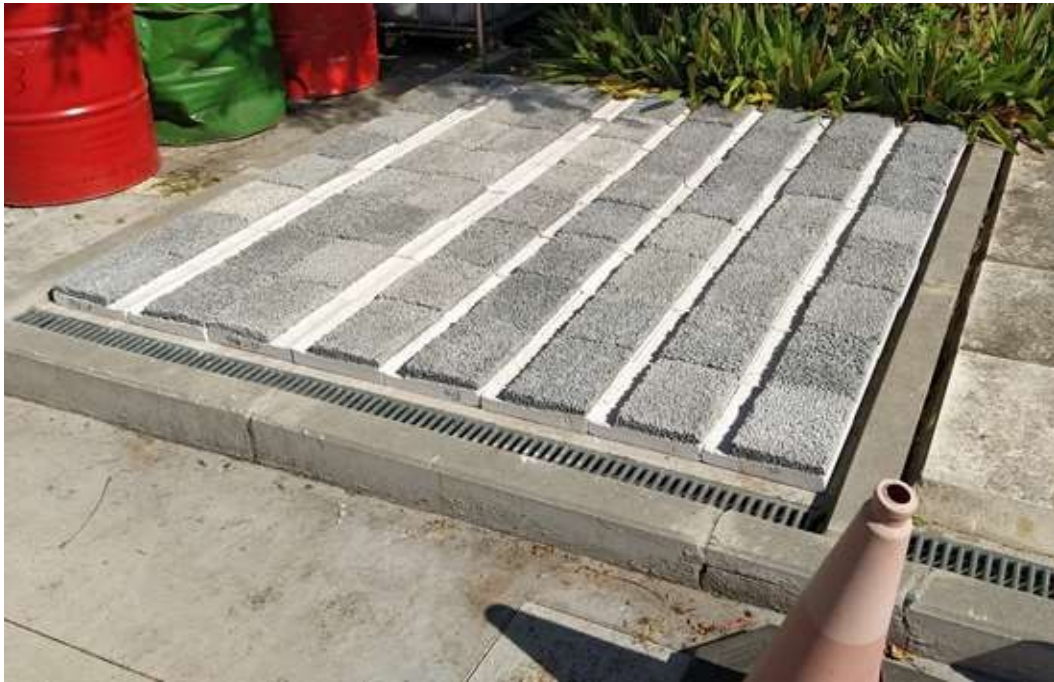
Figure 14: Tiles installed in the IETcc-CSIC facilities.
