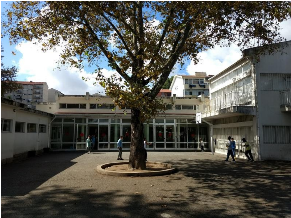
Figure 10. Exterior area in front of south façade F2.
