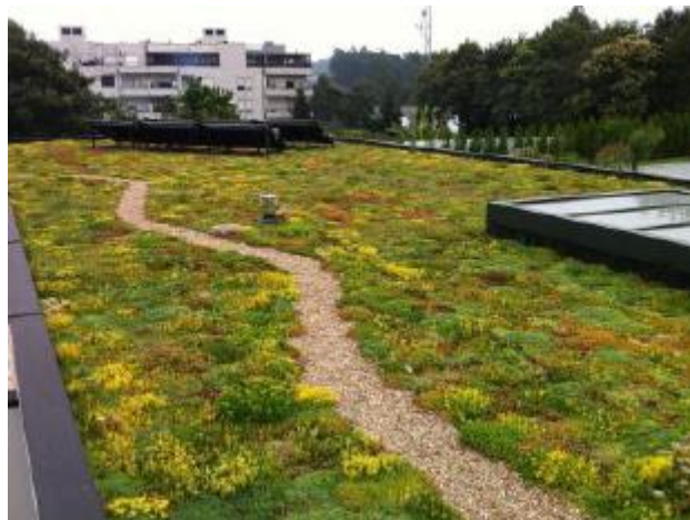
Sedum Carpet in a rooftop. Source: LandLab.
