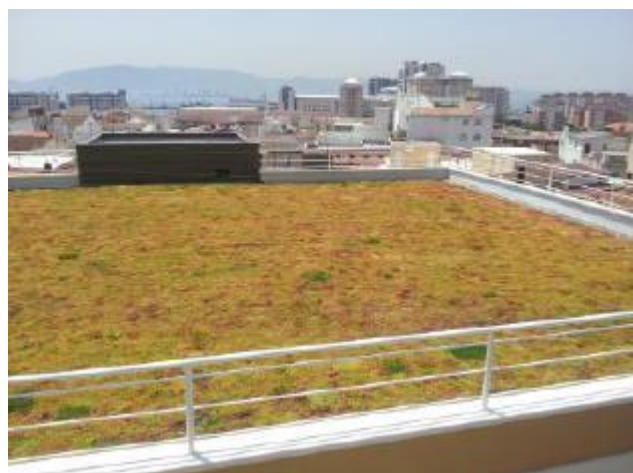
Figure 14. Example of Sedum carpet on a roof. Source: Landlab.
